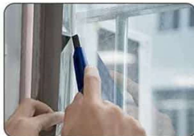
9. Trim away extra film on the edge of the window frame
