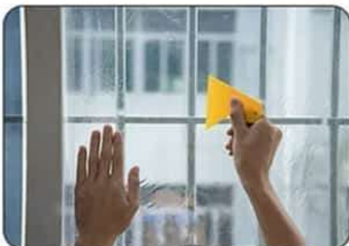
8. Squeegee out air bubbles and imperfections
