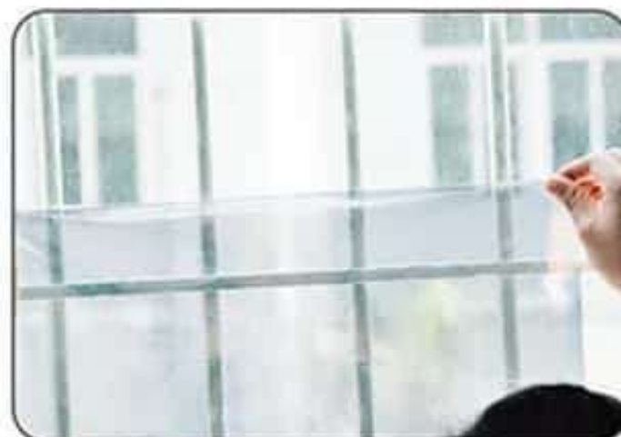
6. Put the film on the window
